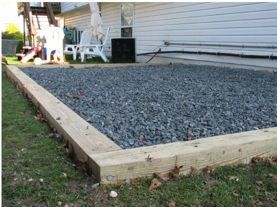
Floor Skid Placement
